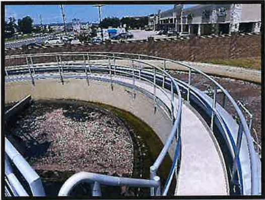
Figure No. 2 – Clarifier Interior
