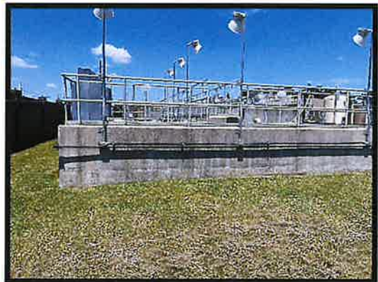
Figure No. 36 – Tank Exterior
