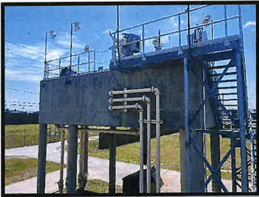
Figure No. 37 – Head Works Exterior
