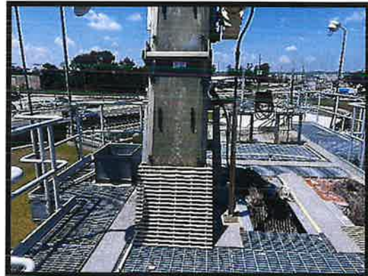
Figure No. 40 – Head Works Screen
