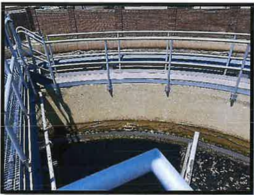
Figure No. 5 – Clarifier Interior
