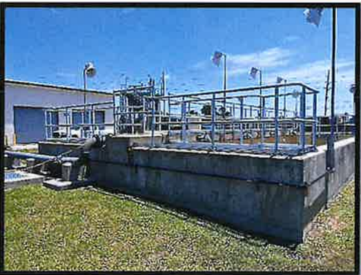
Figure No. 35 – Tank Exterior
