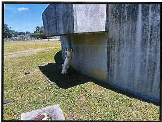
Figure No. 28 – Tank Exterior
