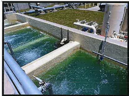
Figure No. 34 – Tank Interior
