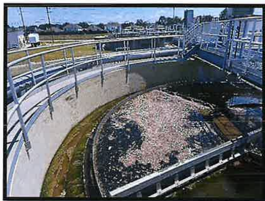
Figure No. 6 – Clarifier Interior
