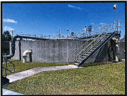
Figure No. 1 – Tank Exterior
