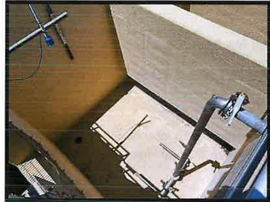
Figure No. 32 – Tank Interior
