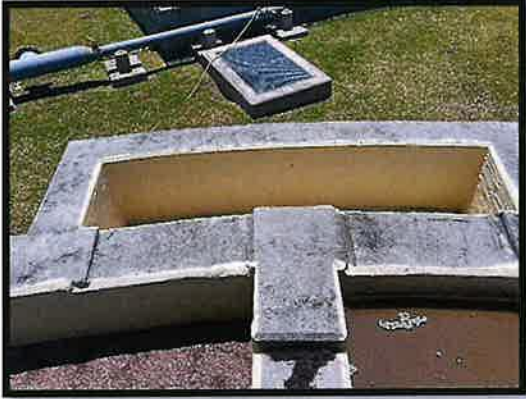
Figure No. 12 – Tank Interior
