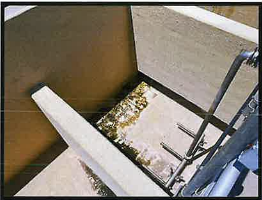
Figure No. 33 – Tank Interior
