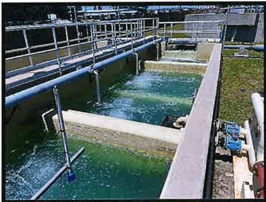
Figure No. 29 – Tank Interior
